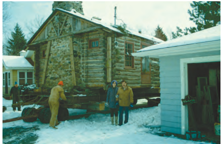
With just inches to spare, the Cabin was eased out from the back yard.
