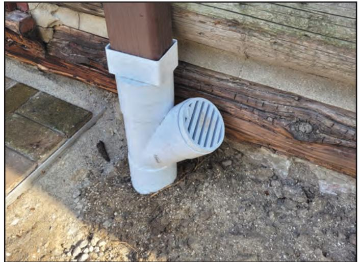
**A trench was dug and two downspouts were buried to drain water to the west of the Cabin.**
