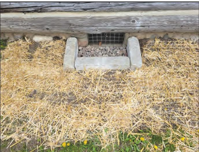
**Weston wall blocks were used to create a window well on the east side of the Cabin.**
