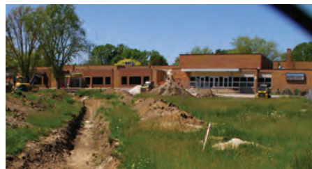
New addition to Hales Corners Elementary School on Janesville Rd.
