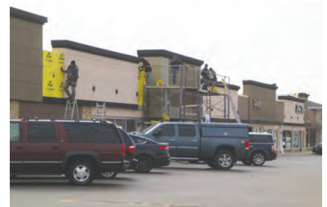
The "Facelift" in progress
